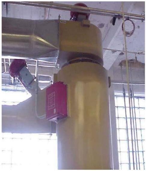
Application of the Isolation System to a dust collector cyclone. The cyclone is explosion protected by an explosion vent that discharges through a short duct to the outside of the building (not shown). The inlet and outlet ducts are protected by isolation cannons to extinguish burning material that would present an explosion ignition risk within the dueling and inside connected equipment.
